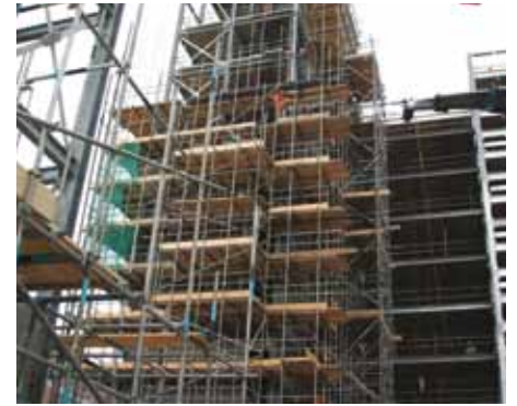
City Centre Carpark
