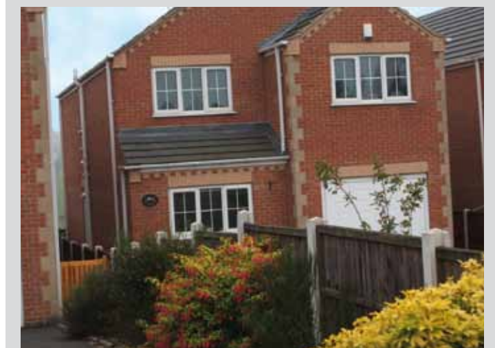
Project: Shuttlewood, Derbyshire 8 No. 4 bedroomed detached houses Value: £1 million Year: 2003/2004
