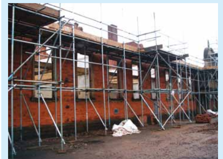
Project: 17 new houses and 2 school conversions Main Contractor: DRC Construction Contract Value: £200,000 Year: 2007/2008
