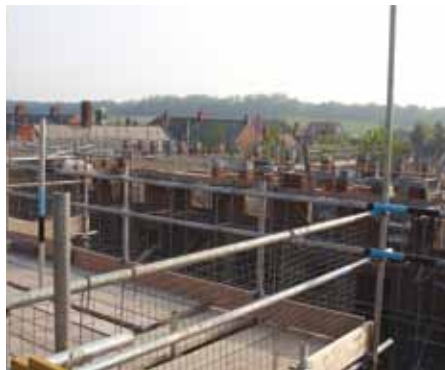
Scaffolding & brickwork combined packages
