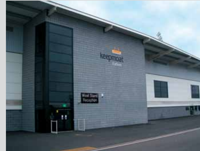
Project: Keep Moat Stadium (Doncaster FC) Main Contractor: Carillion (Civils) Contract Value: £880,000 Year: 2006/2007
