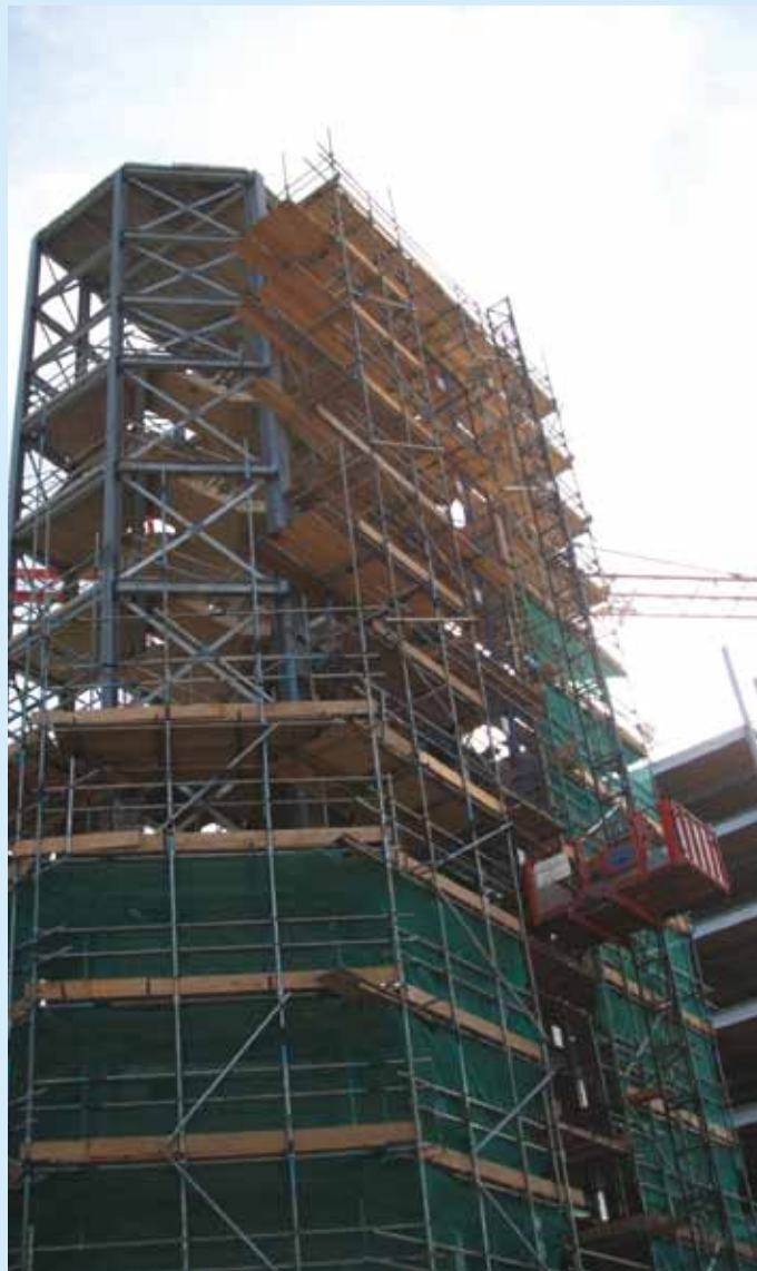
Project: City Centre Carpark Main Contractor: Bourne parking Contract Value: £330,000 Year: 2008
