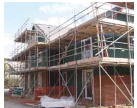
Timber Frame Scaffolding
