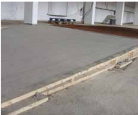
Forming new carpark ramp
