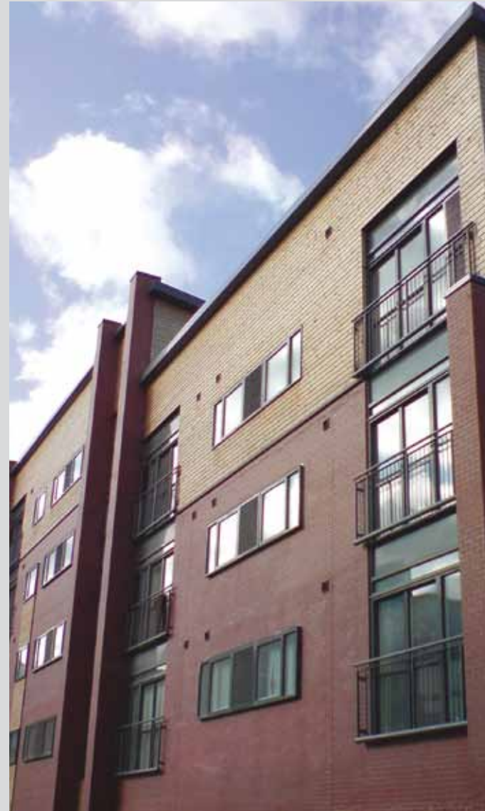
Project: City Centre Apartments Main Contractor: Esharoth Contract Value: £450,000 Year: 2008
