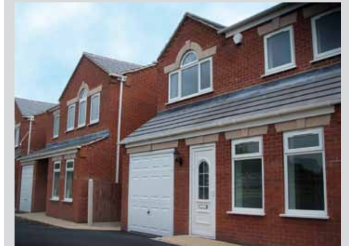
Project: Hardwick View 12 No. 4 bedroom detached houses Value: £2.5 million Year: 2006/2007
