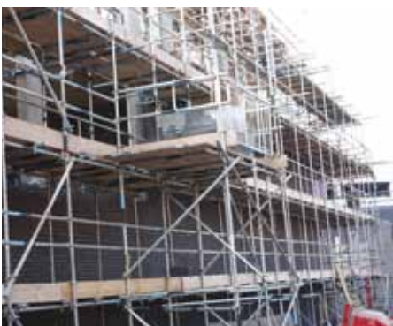
Scaffolding & brickwork packages
